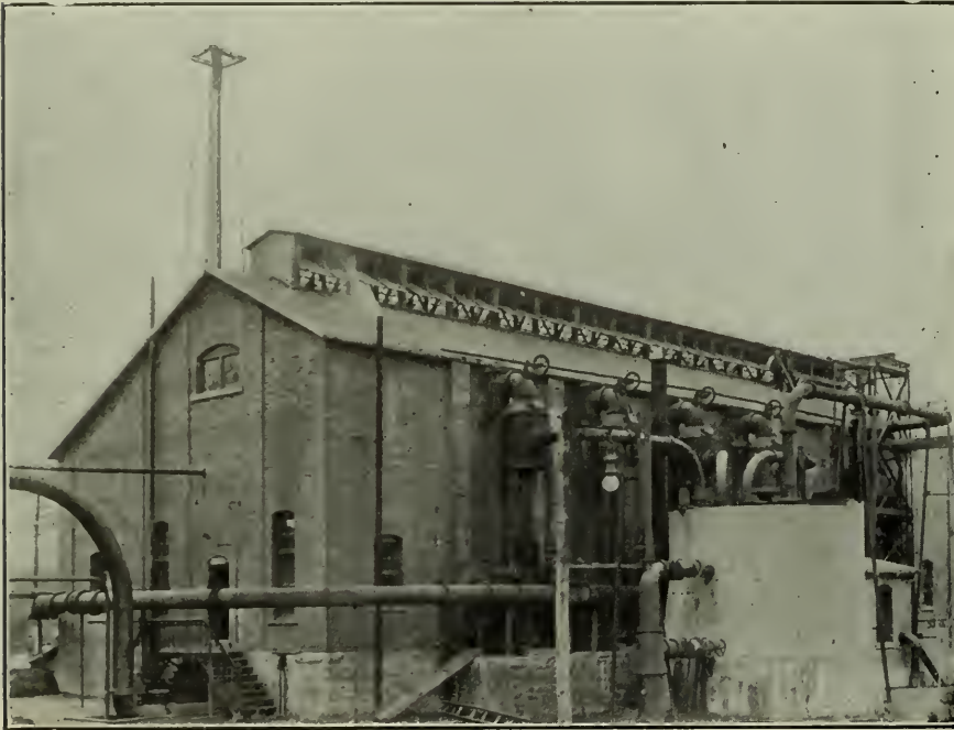
FIG. 11. SHOWING THE BAROMETRIC CONDENSERS
